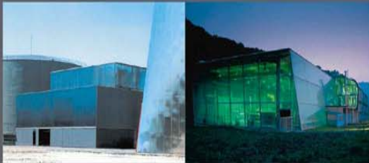
MATE GLASS RESTRROOMS & ROOFS
