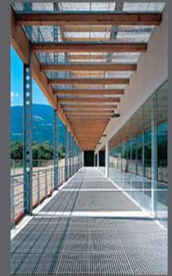
IRON GRILL FLOORING STAIRCASE AND PASSA- GEWAY, FIRST FLOOR
